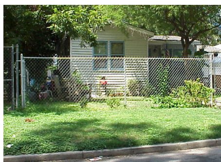
Example of non-conforming fencing material
