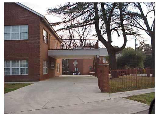
Inappropriate ancillary structure height (background) (same as primary structure, foreground)
