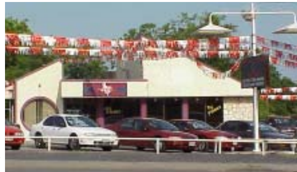
Examples of non-conforming fence material
