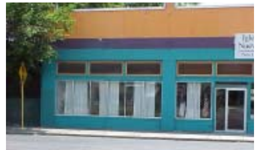
Example of conforming window and door openings on a commercial structure
