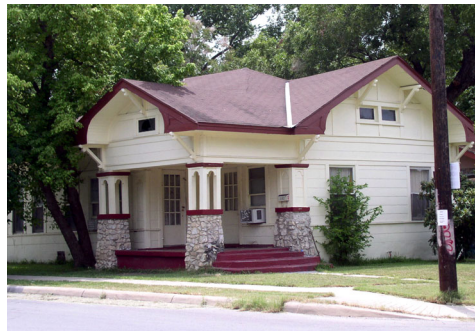
Appropriate use of common building materials
