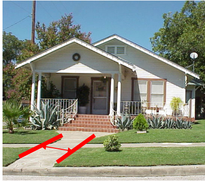
Typical example of front walkway on a residential property; Single-family structures require 36" walkway
