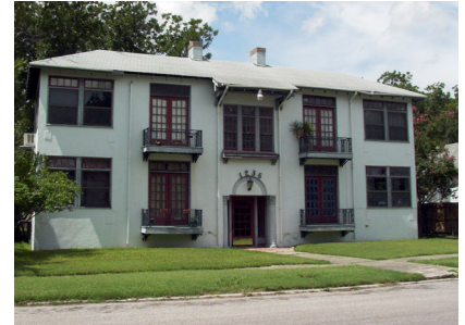
Appropriate window dimension and percentage of first floor dedicated to window openings
