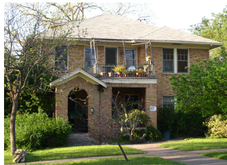
Residential structure with an appropriate porch width (greater than 1/2 of the structure's street façade width)
