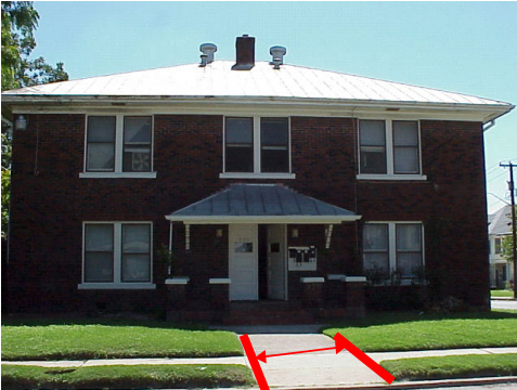
Typical example of front walkway on a residential property; Multi-family structures require 48" walkway
