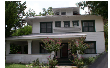
Typical two-and-a-half story residential structure
