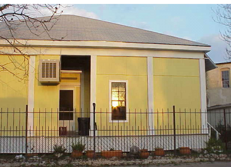
Residential structure with a non-conforming enclosure and transparency ratio of an existing porch
