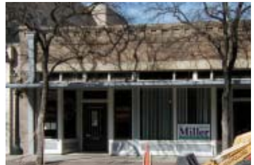
Example of appropriate entrances and door openings
