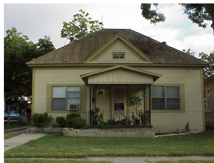
Residential structure with a non-conforming porch width (less than 1/2 of the structure's street façade width)
