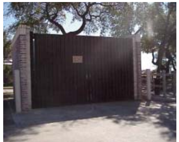
Example of conforming concealed refuse container
